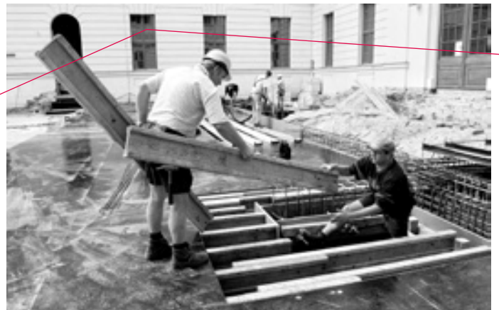
Completing the foundation of the courtyard
